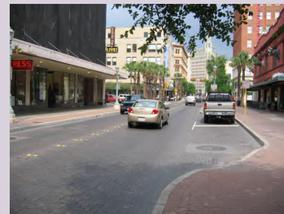
Curb bump outs and striping help better define the parking lane from the travel lane
