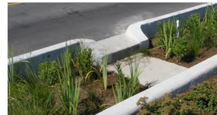
Bioswales treat runoff in Indianapolis
