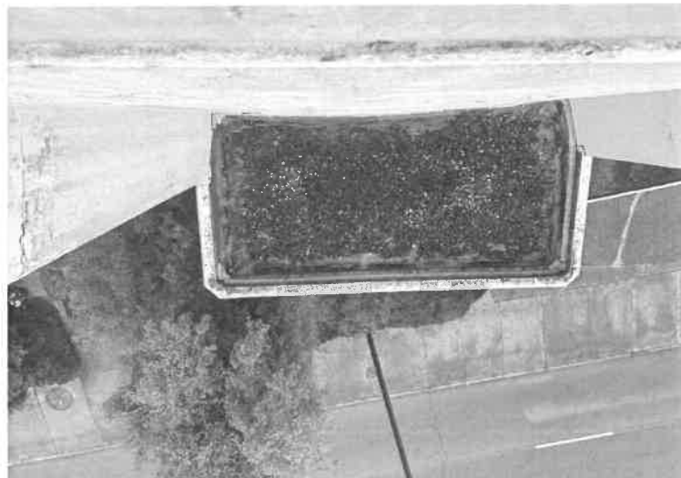
Photo 37: View Looking Down at Top of Entrance Awning
