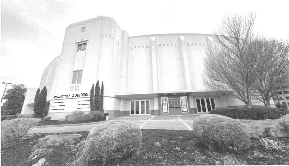
Photo 4: Distinctive Art Deco Facade
