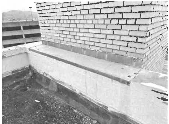
Photo 33: Flashing at Chimney Integration
