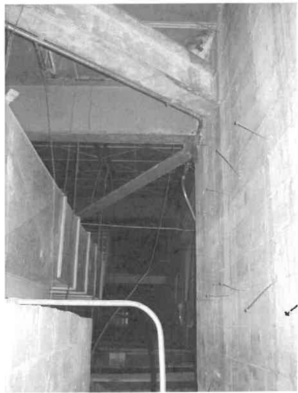
Photo 9: Steel Framing Supporting Ductwork
