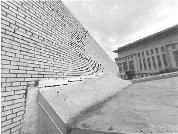
Photo 34: Sheet Metal Integration with Masonry Masonry Wall
