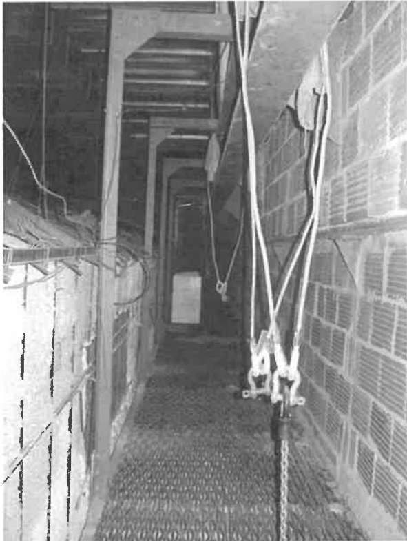
Photo 10: Catwalk Supported by Steel Structure and Clay Tile
