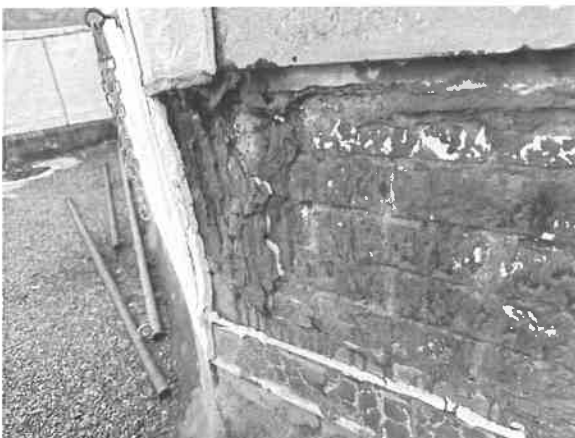
Photo 29: Roof Termination Between Brick Masonry Wall and Concrete Façade
